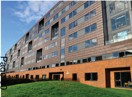
Horizontal seamed cladding with recessed or projected bay windows to articulate the elevation
