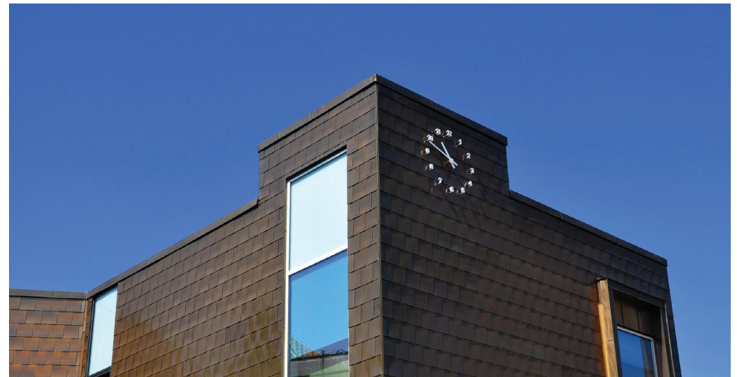
Example clock face on brass shingle cladding
